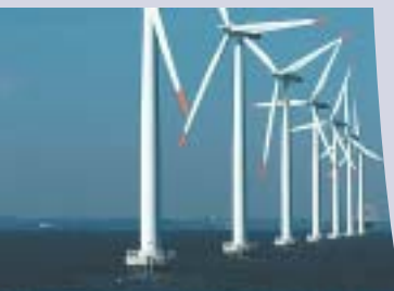
Offshore wind farm
